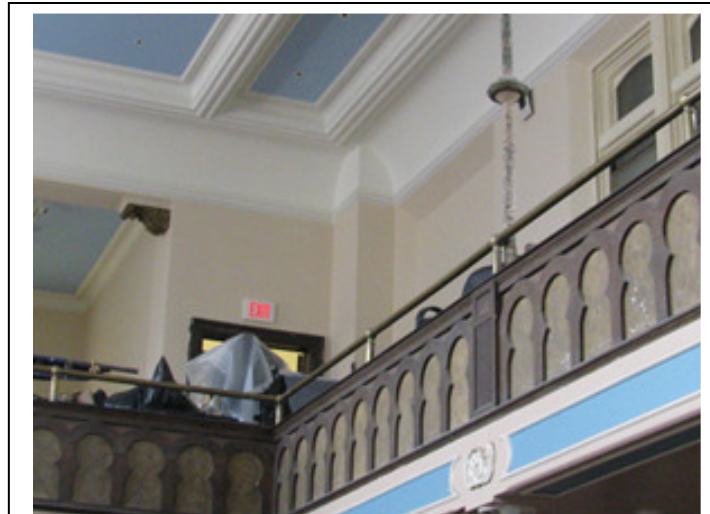
Repaired plaster and a first coat of paint in the balcony Photos courtesy of Ken Schept
