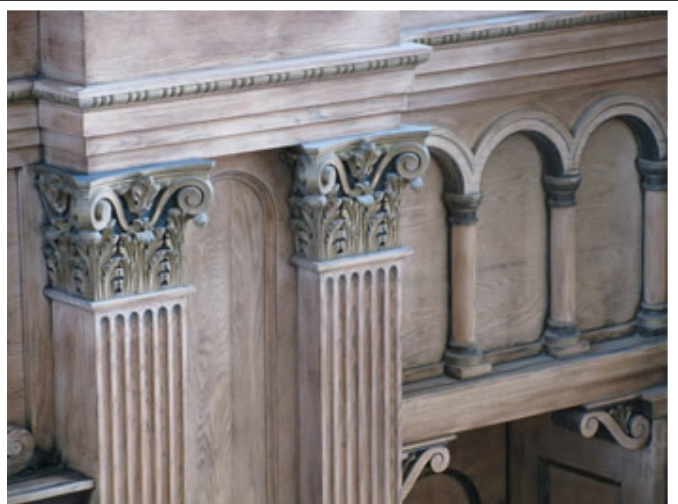
Detail of the Ark Wall, after stripping
