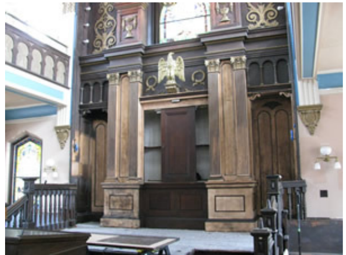
Early stages of stripping the ark wall (June 25)
